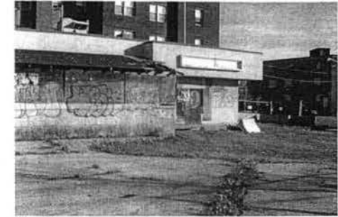
Vacant/boarded up property at Quncy Street/Georgia Avenue
